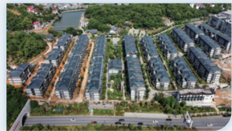
Pengnan Company's Photovoltaic Floodlighting Project
