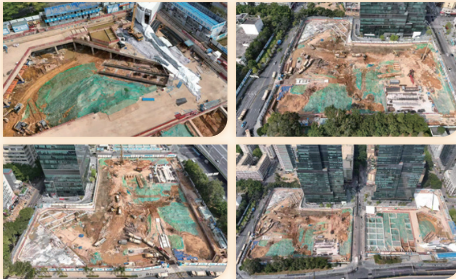
Phase II of Chegongmiao First Revitalization Project
