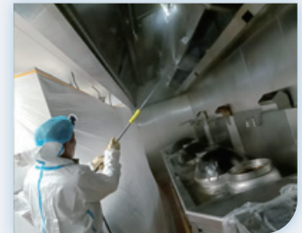
Commercial Management Company's Exhaust Duct Renovation
