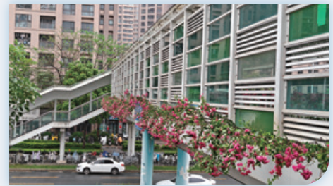
“Air Corridor of Flowers” Revitalised Urban Footbridges
