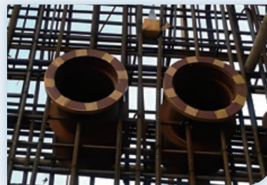
Installation Site of the Flexible Waterproof Casing for the Three-stage Water Stop Casing
