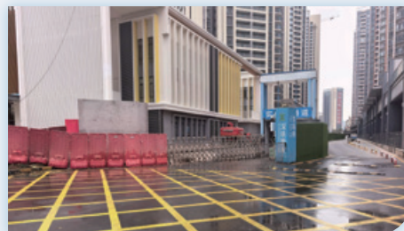
Ground Washing for the Constructing Section
